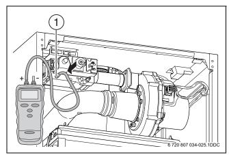
Fig. 45 Connecting the pressure gauge at type 100
