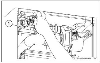
Open the burner pressure nipple at the type 100 Fig. 43
