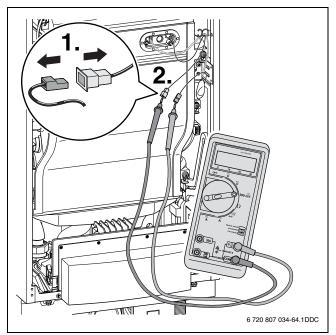
Fig. 49 Connecting the multi-meter
